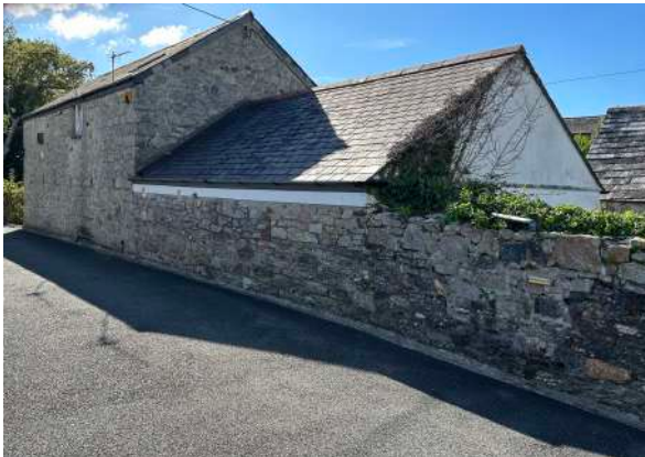
Photograph 1. South and east elevation.
