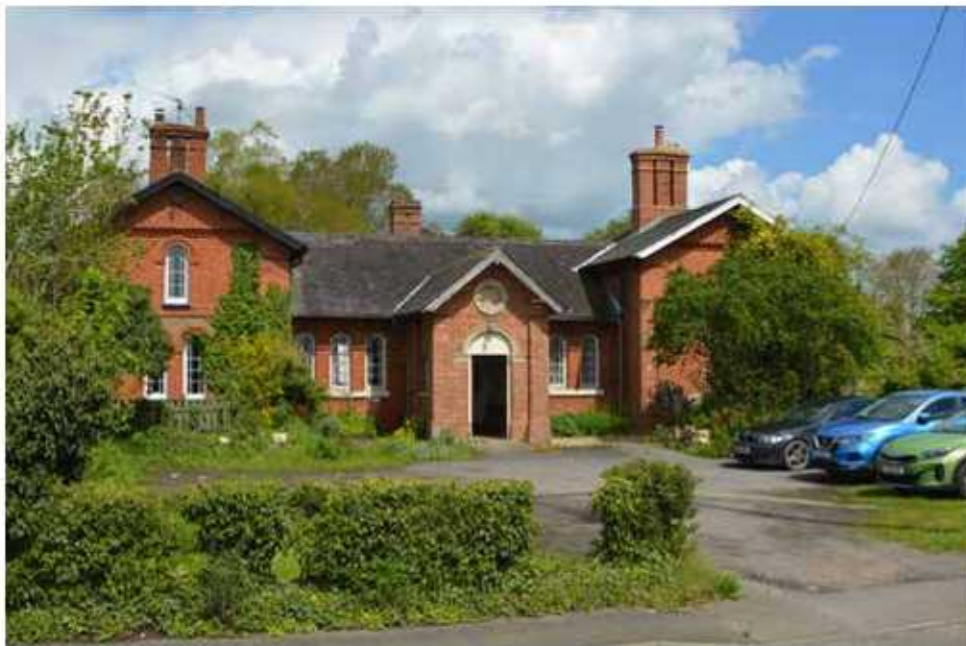
Above: Photograph taken from main road of front elevation, facing north.
