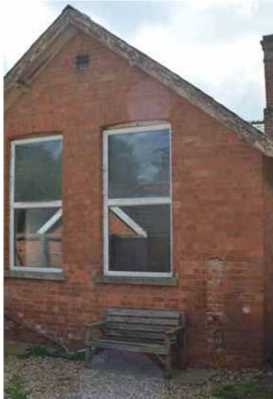
Above: external rear north elevation, gable end.
