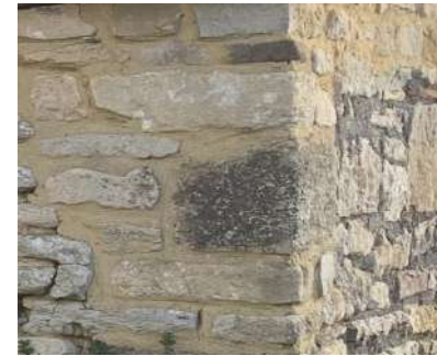
FIG 30. EXISTING RUBBLE STONE RETAINED, PROPOSED EXTENSION STONE TO MATCH.
