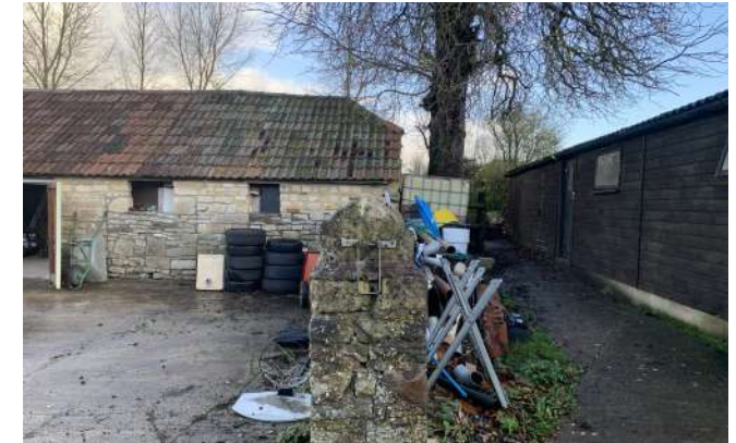
FIG 3. LOW-LEVEL STONE WALL
