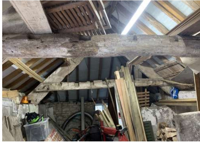
FIG 47 Barn interior, looking west. Original and later structural timbers are visible
