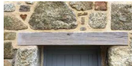
FIG 31. TIMBER LINTELS
