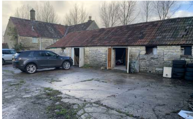
FIG 2. EXISTING BARN EXTERIOR, SOUTH ELEVATION
