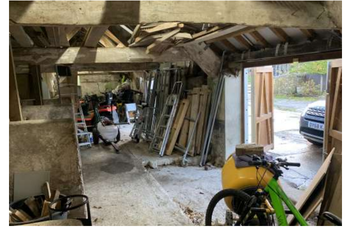
FIG 49 Barn interior, looking east, access doors to southern aspect hardstanding. Main trusses and stepped concrete floor visible.
