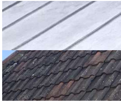
FIG 27. METAL SHEET / CLAY TILES REUSED WHERE POSSIBLE.
