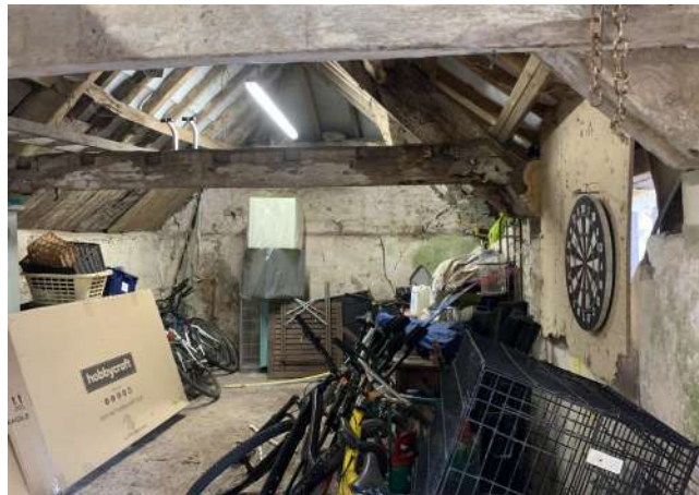
FIG 48. Barn interior looking east.
