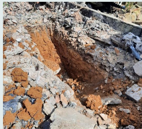
Concrete over gravelly Made Ground and clayey Head in TP5
