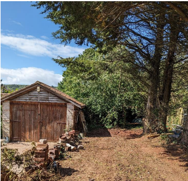
1.04 Eastern Elevation of Builders Store
