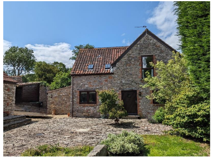
1.12 The Residential Annexe for The Coach House
