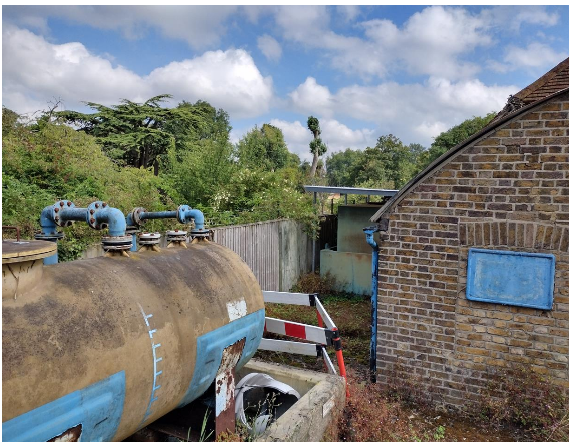
Photo 2: Fuel tanks adjacent to Luxmores Garden
