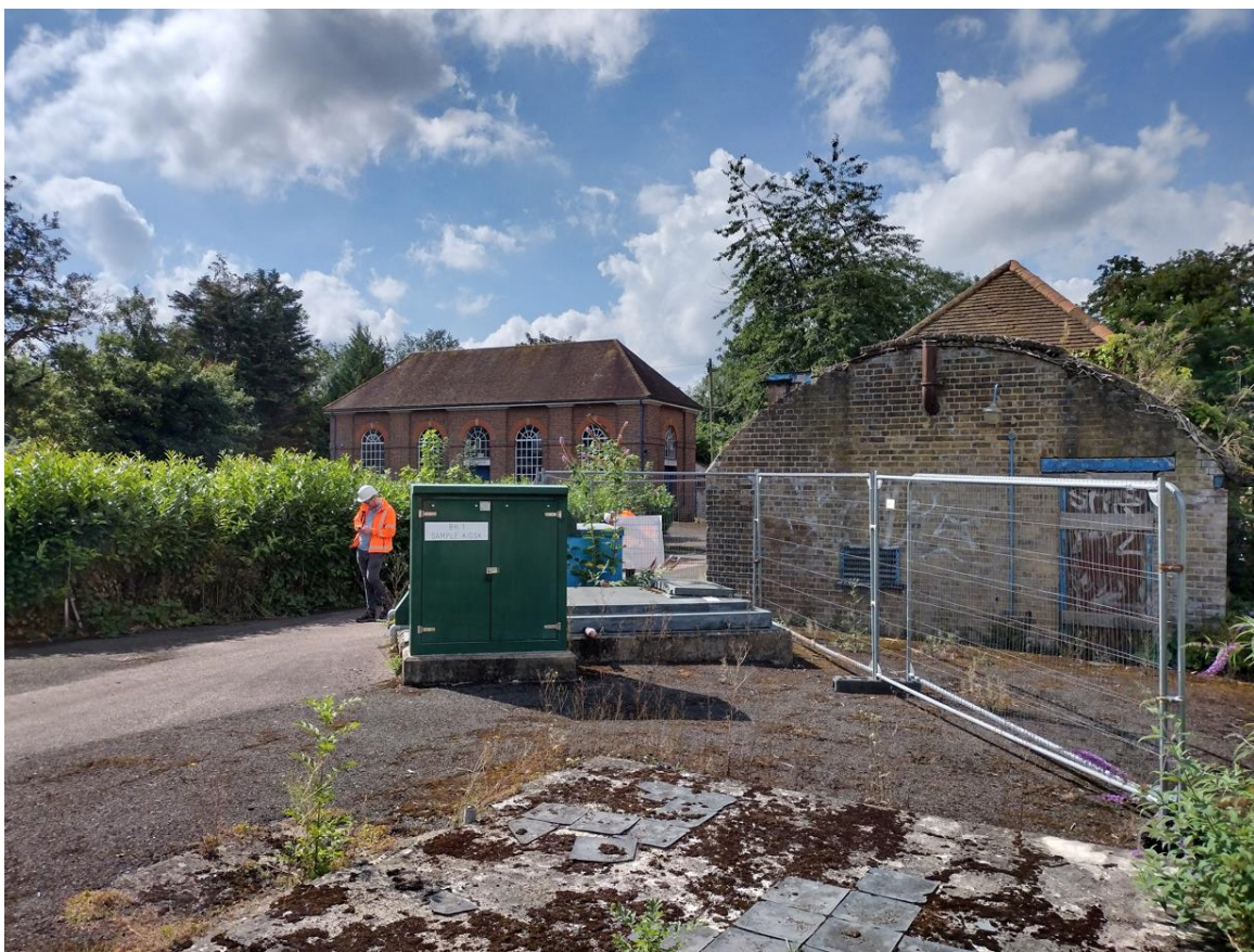
Photo 4: Northeastern elevation and view towards filter house
