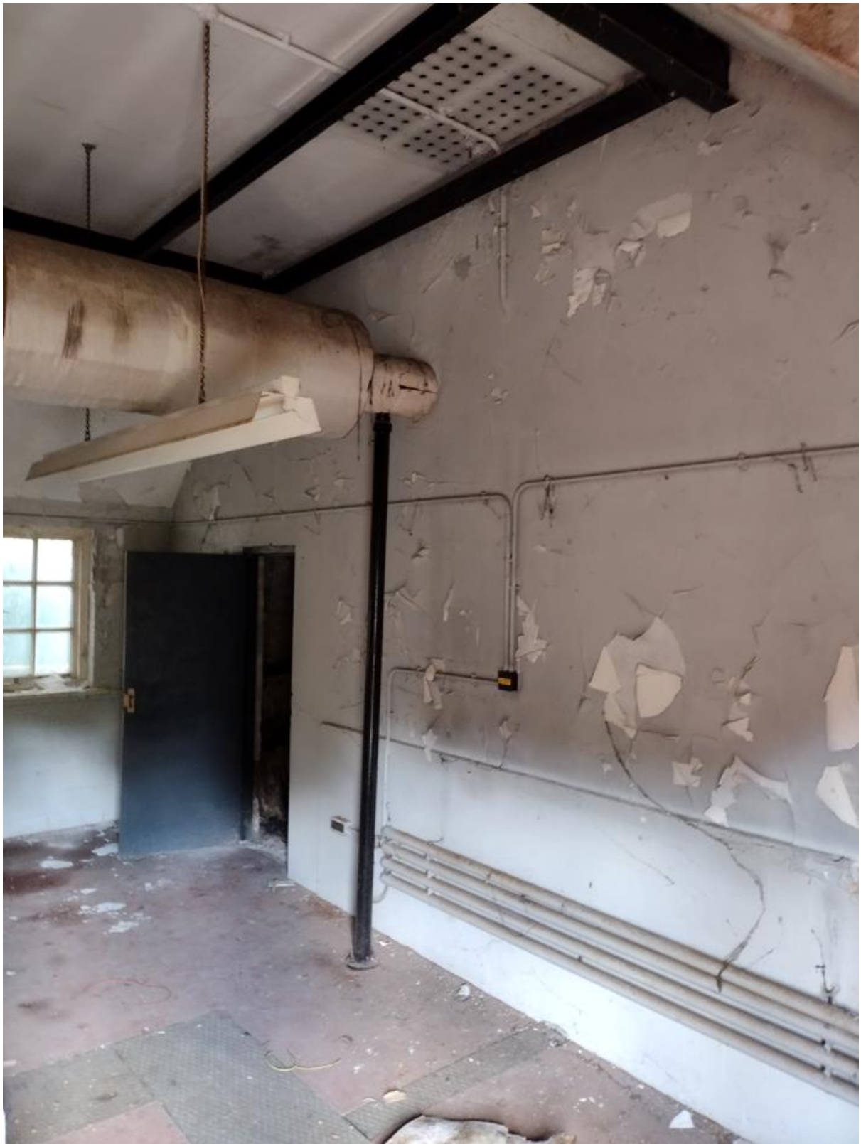
Photo 7: Interior of building.
