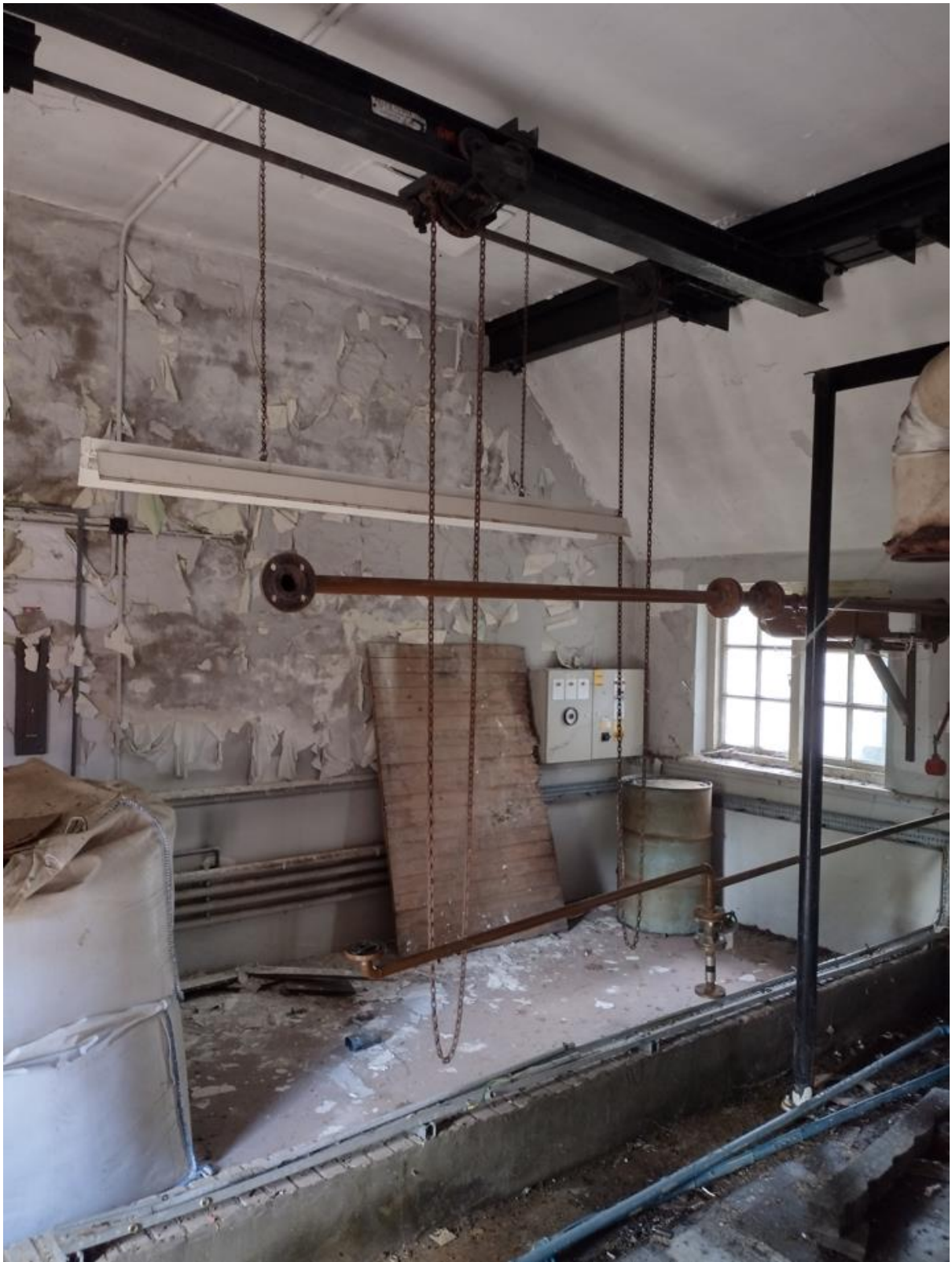
Photo 6: Interior of building
