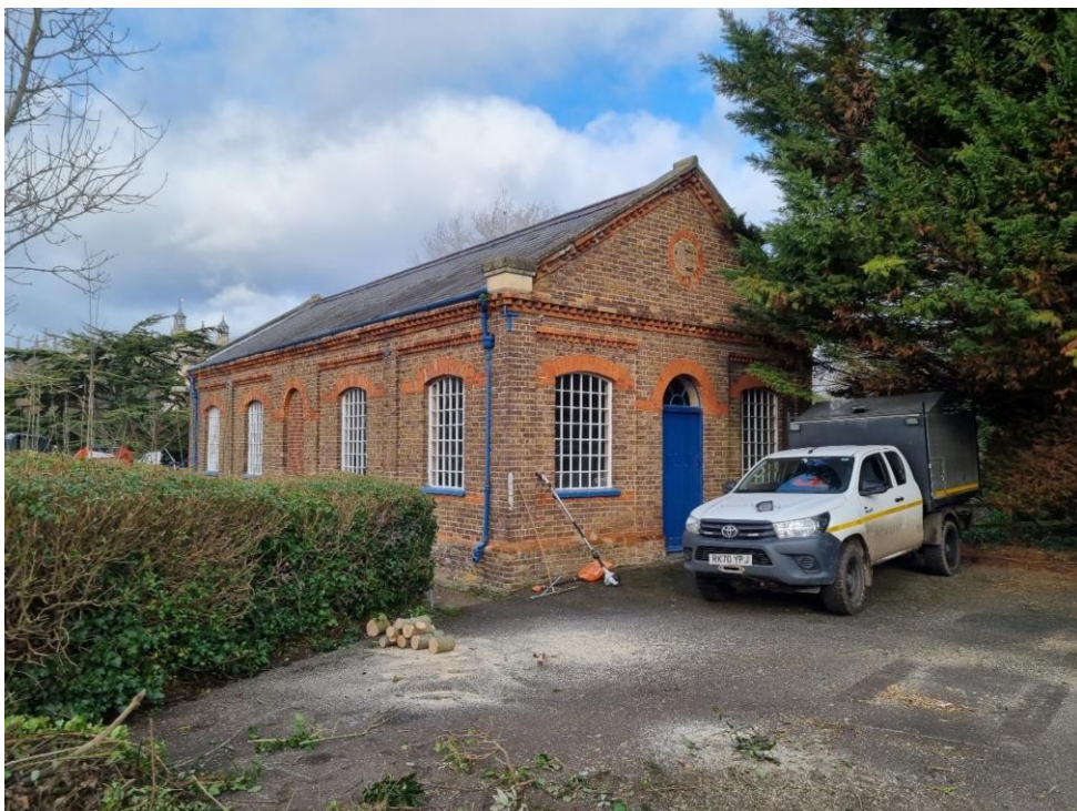
Figure 15: West Pump House
