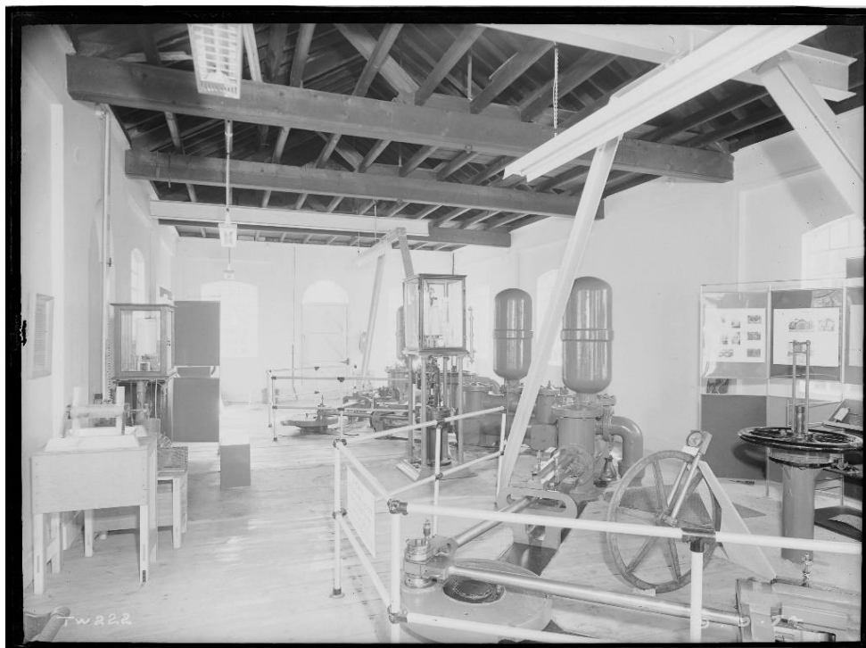
Figure 32: 1974 Archive photo of Pump House I.
