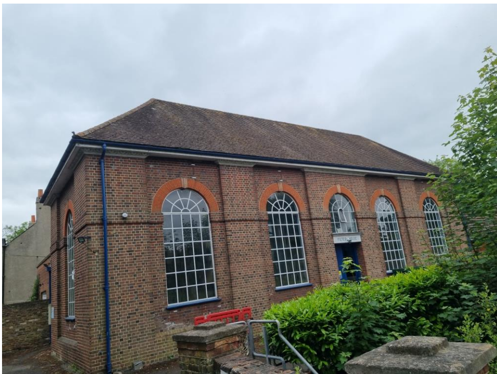
Figure 17: Filter House Building
