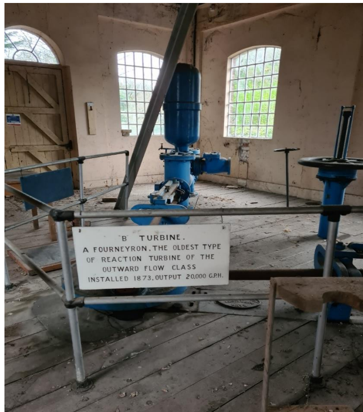
Figure 31: Significant Pump Houses with Fourneyron turbines.
