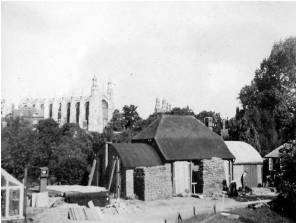
Figure 20: Generator Building September 1939. Sandbagged in preparation for air raids. Chimney visible to northern side that is no longer present. Not clear if concrete covering installed. No extension to front elevation.
