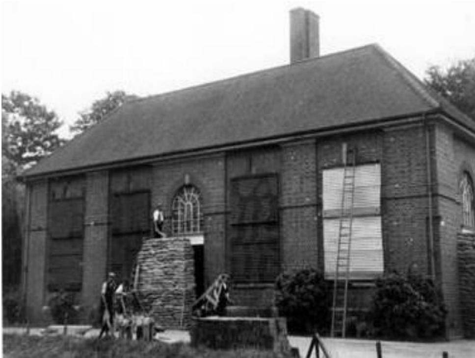
Figure 33: Filter House 1939 archive photo. Being protected from air raids with sand bags and shutters.
