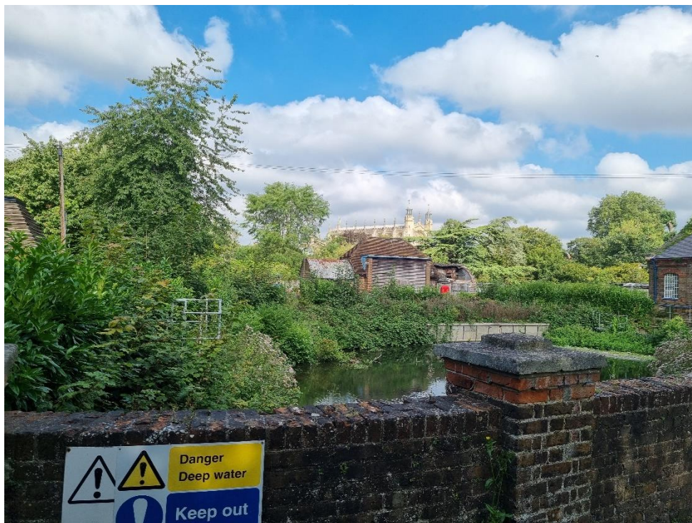
Figure 24: Generator Building with mill stream to front and Eton College in background.
