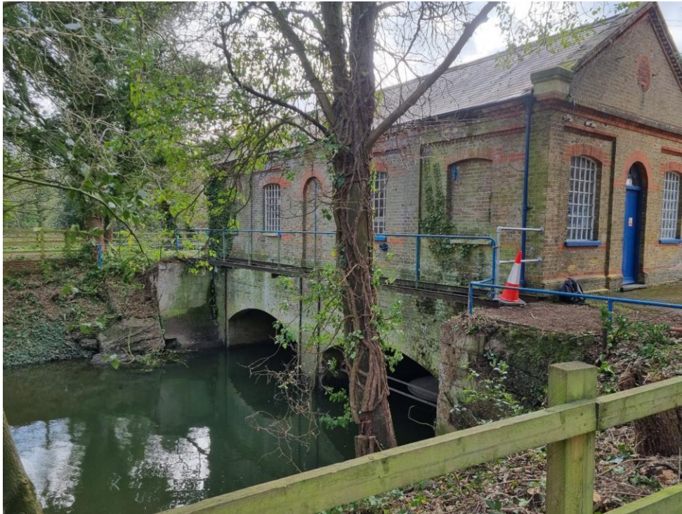
Figure 16: East Pump House
