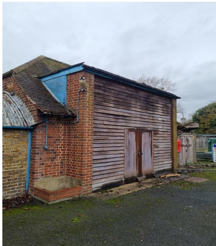
Figure 28: More recent front extension to Generator Building.
