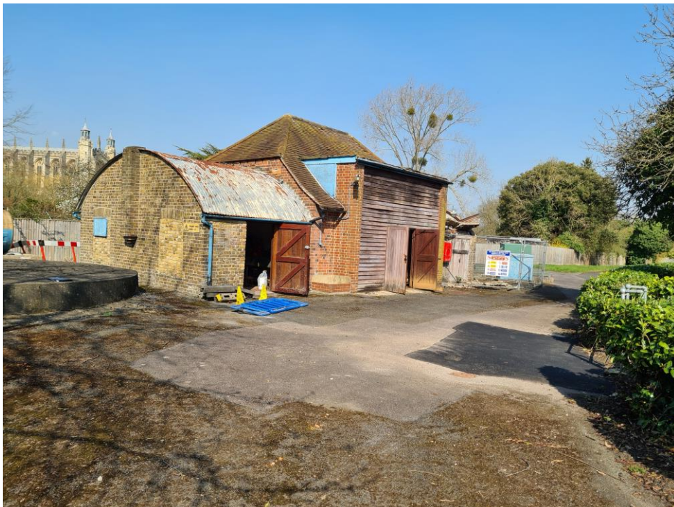
Figure 4: Generator Building. Eton College seen behind.
