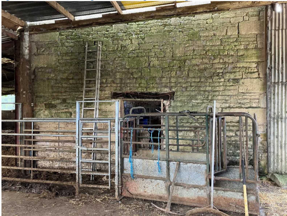
Figure 3 - Rubblestone walling
