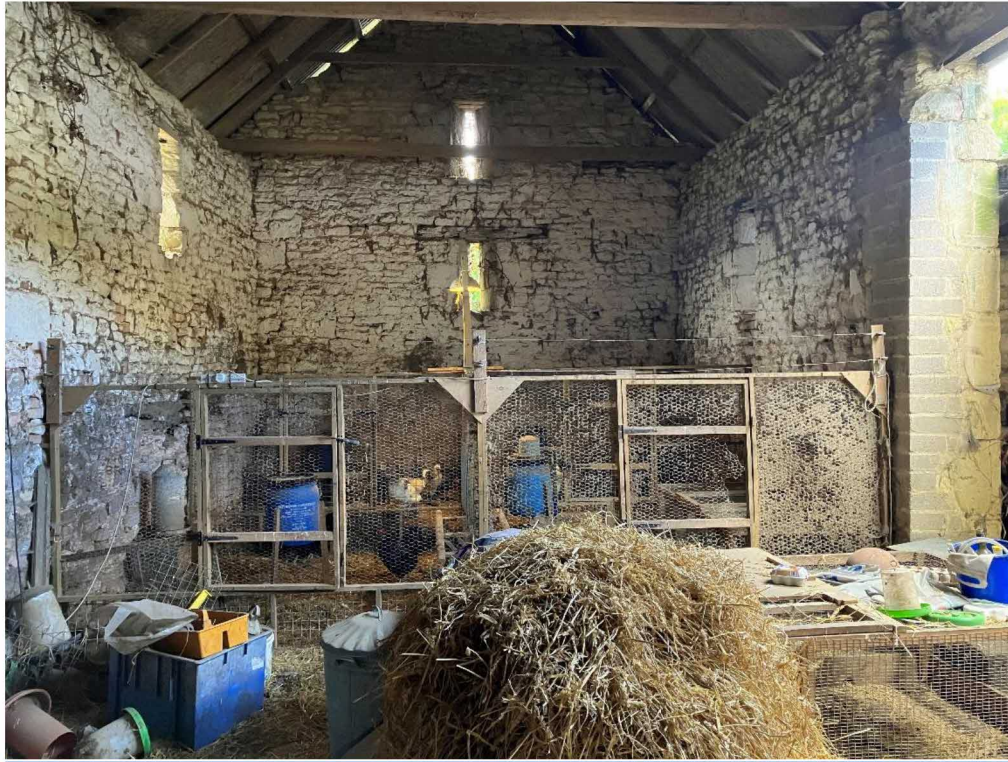
Figure 6 - Internal view of rubblestone walling in main barn
