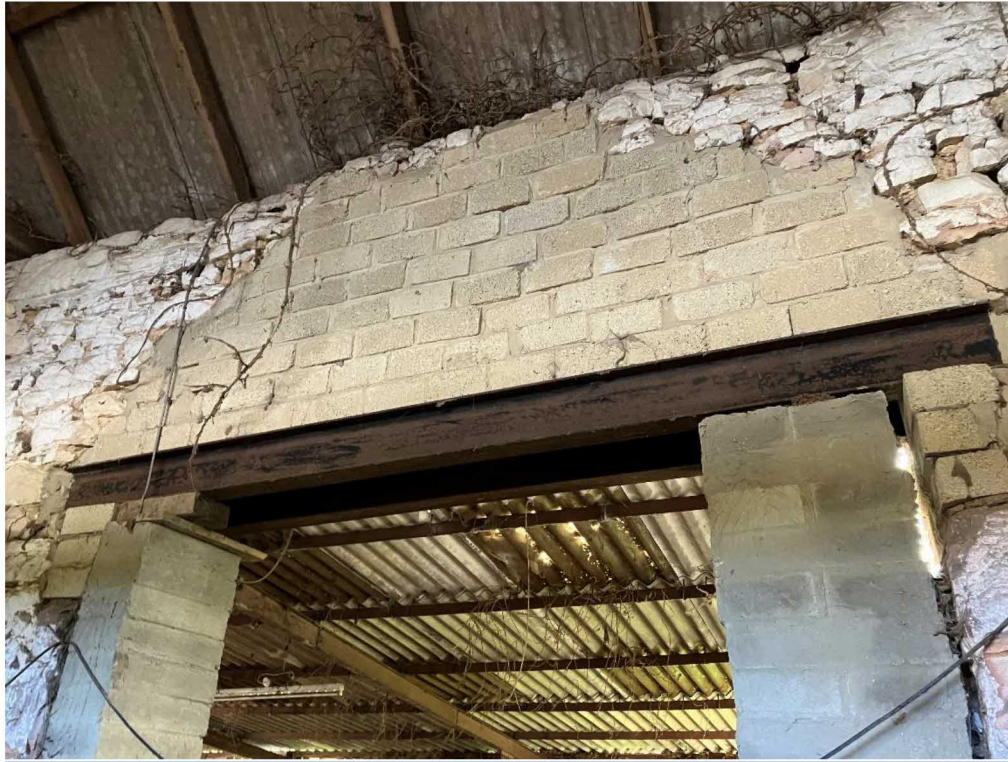
Figure 5 - Historic steel beam sat on pad with more modern walling addition above
