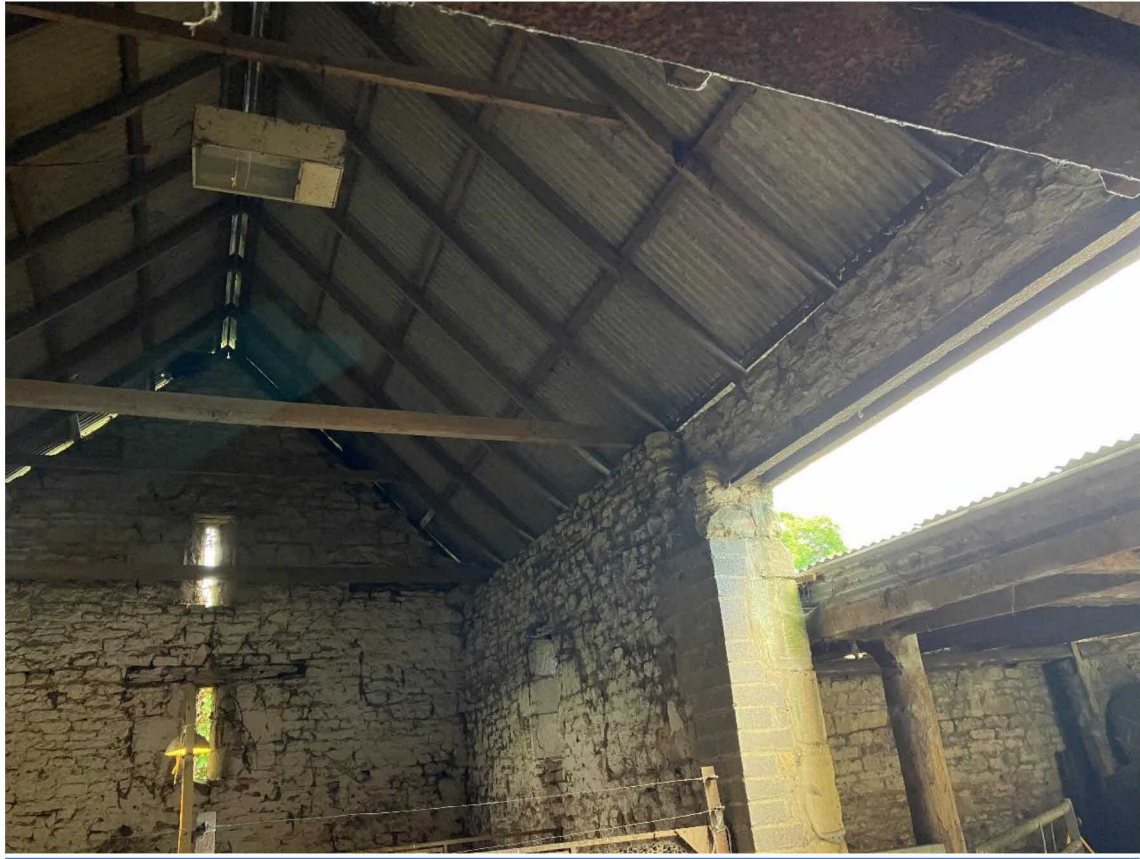
Figure 7 - Internal roof structure / timbers of main barn
