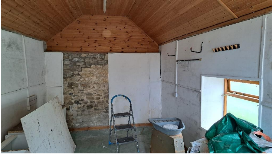
Photo 5 – Internal view looking toward rear.
