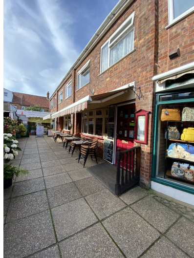
1. Front view of 44c/d Station Road
