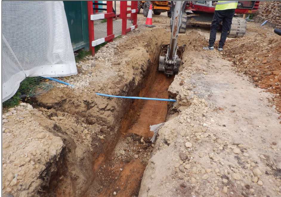
Plate 3. Drainage trench during excavation, looking south
