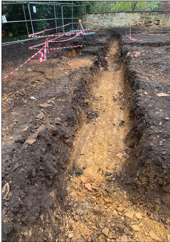
Plate 1. House plot 1, looking northeast
