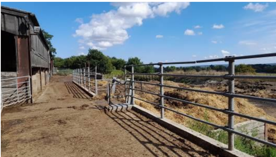
Image 1 – Scrape Ramp, High Dry Matter Slurry Store and Strainer Box
