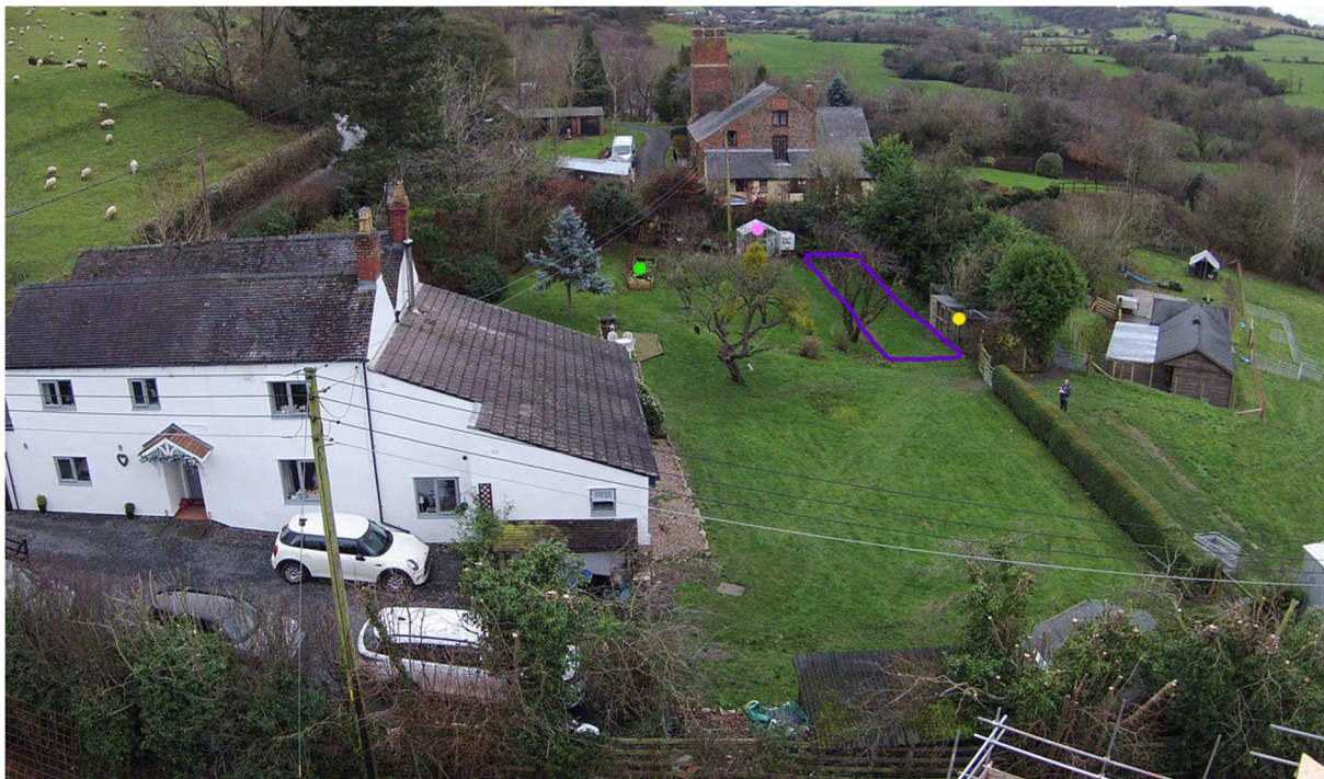
Mistletoe Cottage in December 2018 (exhibiting little change since aerial images of 2010 / 1999) Note especially orchard trees, Greenhouse (●), raised planters (●), domestic cattery (●) proposed hardstanding location (●)
