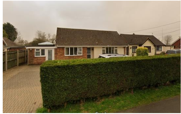
Front elevation of main property
