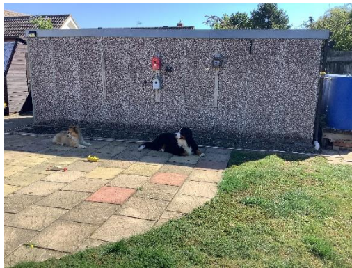
Existing building to be removed (rear garden)
