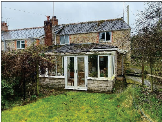
Plate 5: Rear of property and location of proposed works (facing south-west)
