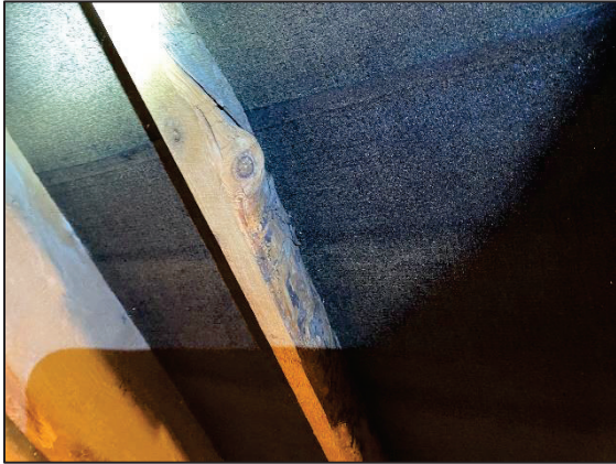
Plate 3: Underside of roof
