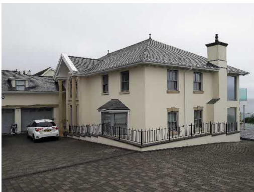
Figure 1 West corner of the building
