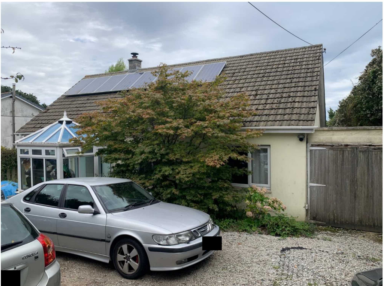
Figure 1: Western Elevation of Building Assessed
