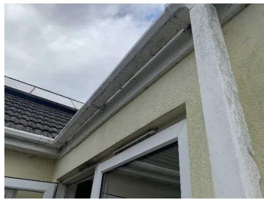
Figure 3: Well sealed fascia, flat roof extension
