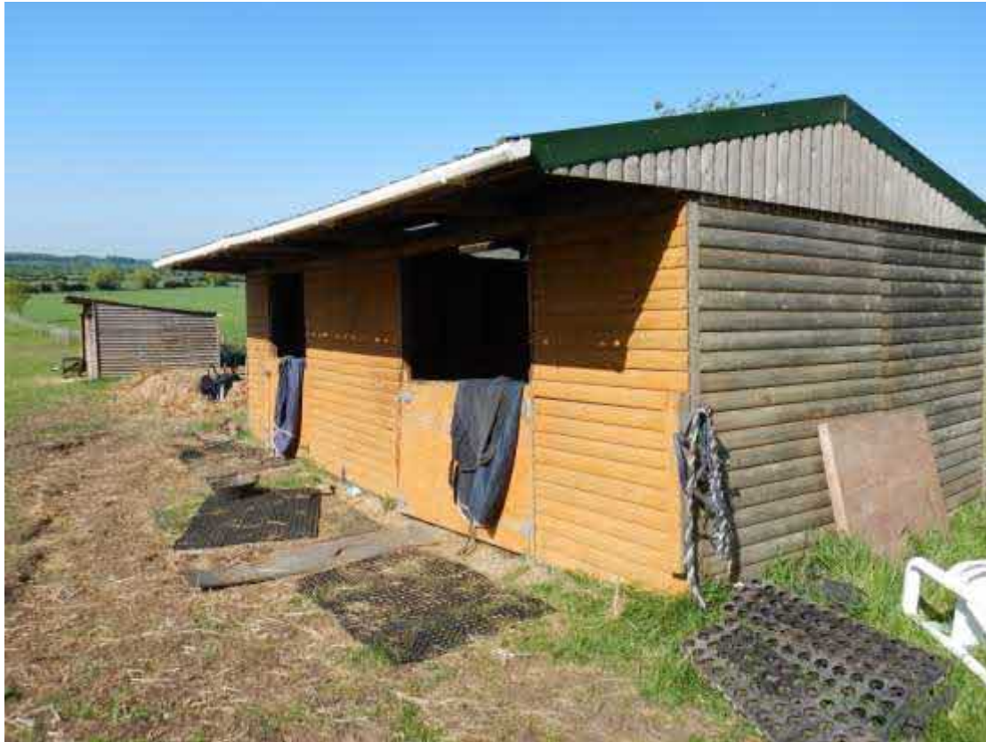
Photograph 8 – The temporary stable buildings that lie outside of the development boundary but within the south-eastern section of the ownership boundary.
