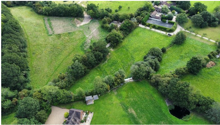
Aerial image from West
