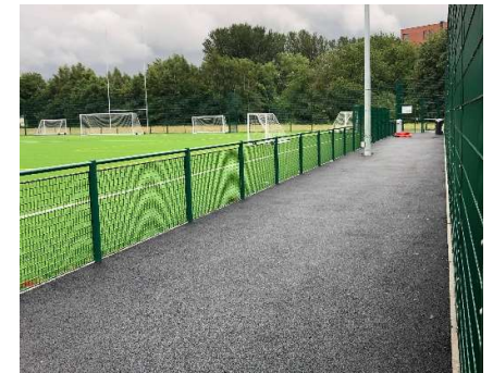
Porous macadam hardstanding to side of pitch
