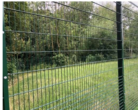
Rigid panel ballstop fencing to perimeter of facility, powder coated dark green so discrete against a rural backdrop
