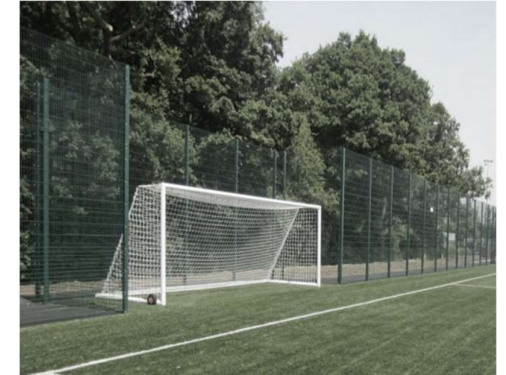
Rigid panel ballstop fencing to perimeter of facility, powder coated dark green so discrete against a rural backdrop
