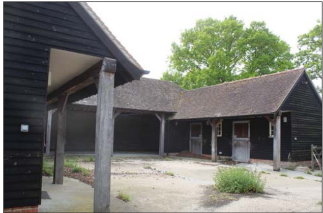
Plate 6. Southernmost stable block, looking south-west.
