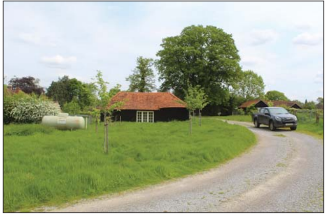
Plate 2. Small building north-west of development site, looking south-east.
