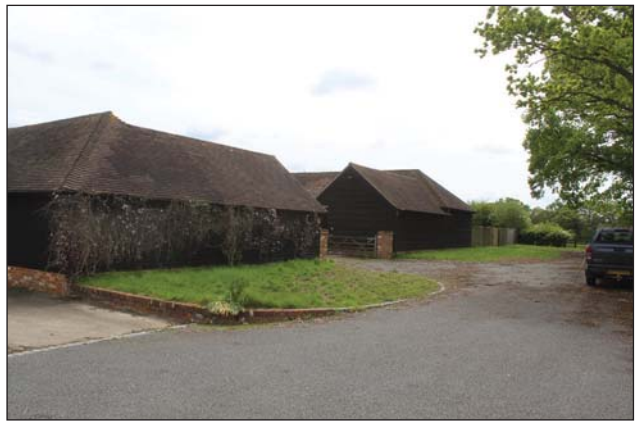
Plate 4. Stable block from trackway, looking south-east.
