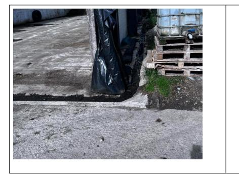
16. Image to show channel drain at permiter of the silage storage area, in place to capture and manage pollution.
