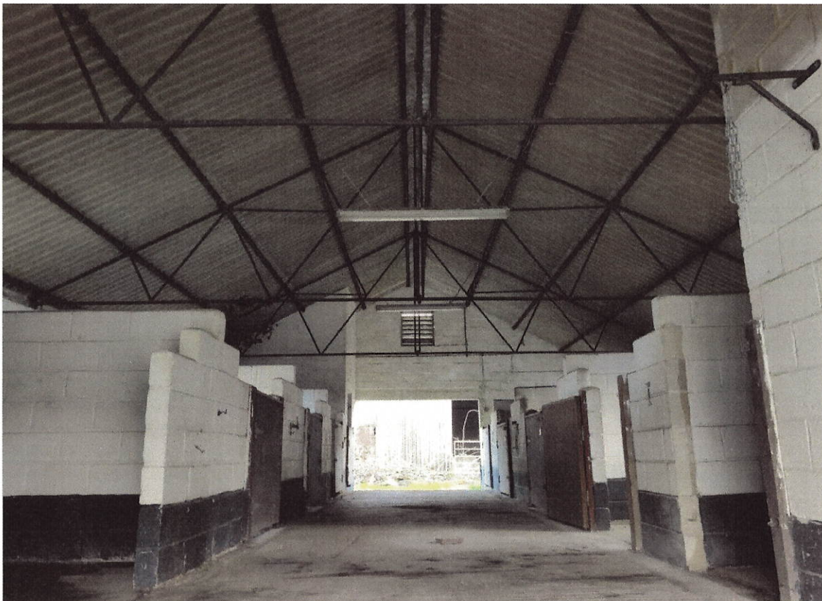
Figure 6 – Internal view looking NE
