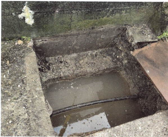
Figure 4 – Trial pit at SW
