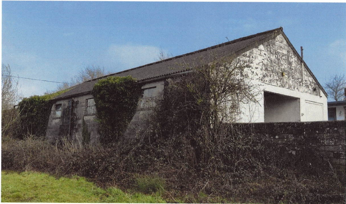
Figure 3 - View from the NW
