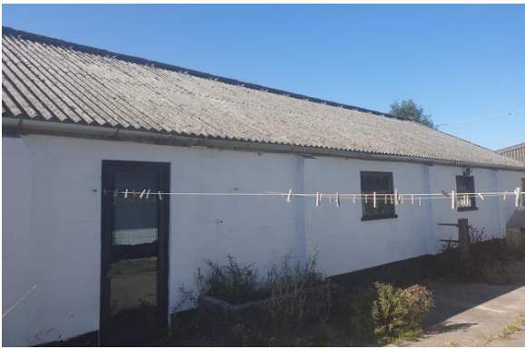
Photograph 7: Cement Fibre Roof
