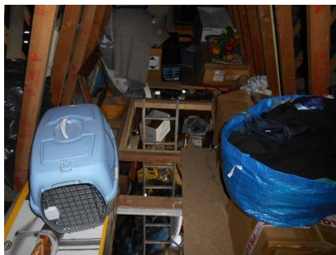
Plate 5: Loft Space Partial Floor
