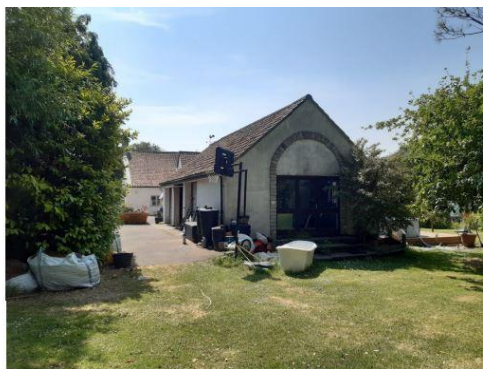
Site Photo 02. Existing North and East elevations of garage viewed from garden.
