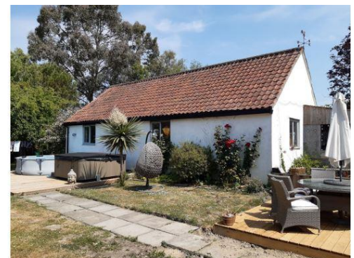
Site Photo 03. Existing West and South elevations of garage viewed from patio area to garden.
