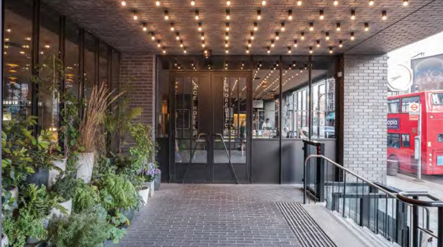
Brick Award Winner Best Refurbishment & Renovation project, Ace Hotel in Shoreditch with Ketley Staffs blue bricks and brick slips
