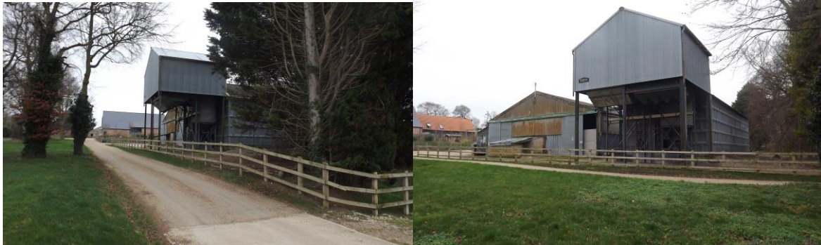
Figure 6 – View of elevated grain hopper feeding into grain dryer B2
