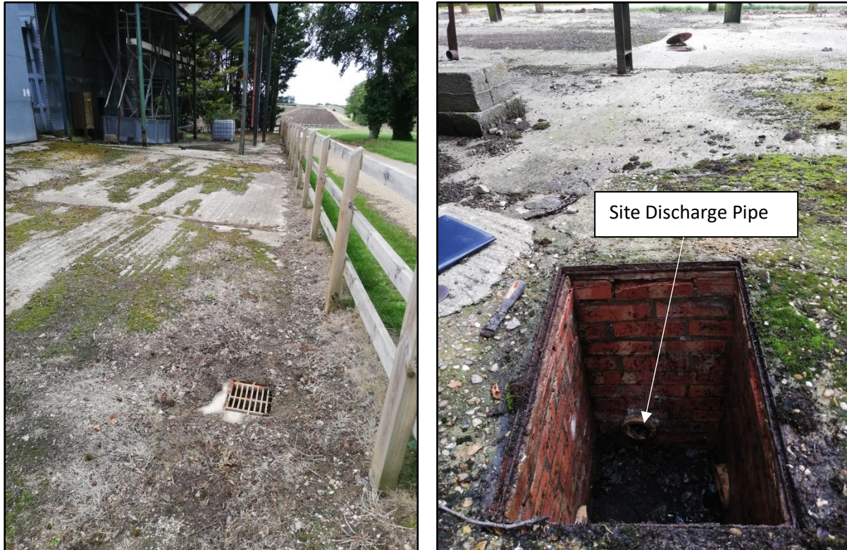
Figure 2 – Existing Site Drainage System
