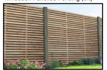
Wooden panels supported by vertical concrete posts with concrete kicker boards (not shown)
