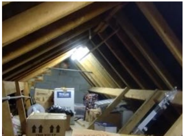
Image 4: Internal view of the main void.
