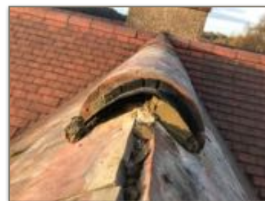
4. To ensure the three ridge tiles remain linked either; place a broken tile over the ridge and mortar only above the tile (left) or fill one side with mortar and leave the other side empty (do this on alternate sides to ensure the feature does not become draughty) (right).
