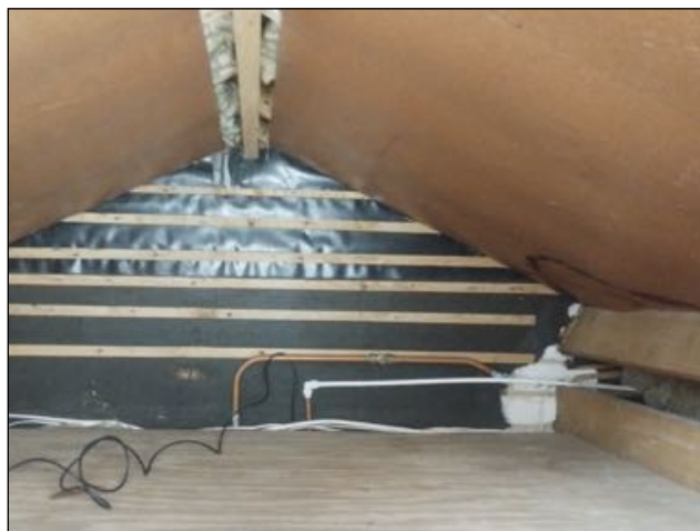
Image 5: Internal view of extension void.
