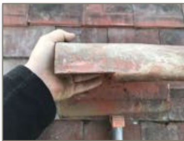
1. Notch out the underside of a ridge tile measuring 20mm high by 50mm wide.
