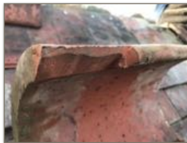
1. Notch out the underside of a ridge tile measuring 20mm high by 50mm wide.
