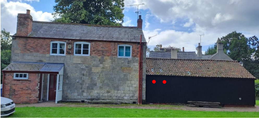
Image 1 – Northwest elevation of Little Cottage with adjoining stables, red circles to indicate proposed boiler flue site (photo taken from proposed site of oil tank)
