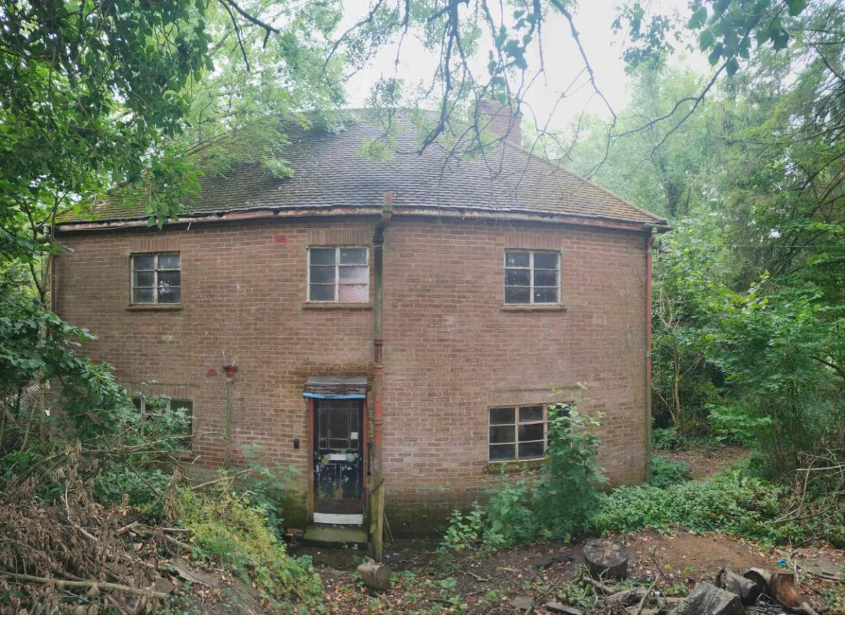
Photograph 5: Existing dwelling from the north
