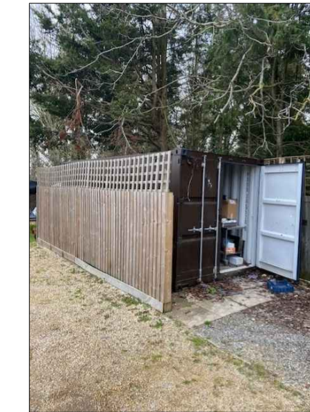
'D' - CONTAINER 6.0m x 2.5m x 2.6m high Screen, 1.8h close board with trellis, 2.4m total height
