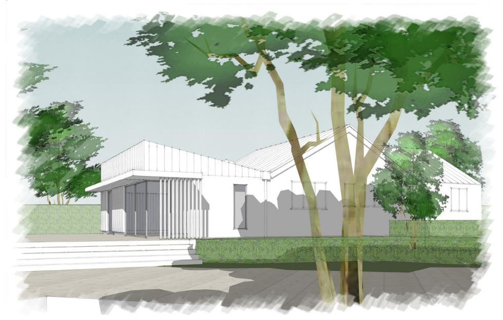
The replacement rear extension features a mono-pitch roof, elevating towards the views over The Fleet and neighbouring fields. New sliding doors improve the connection with the garden and a brise soleil canopy prevents overheating.
