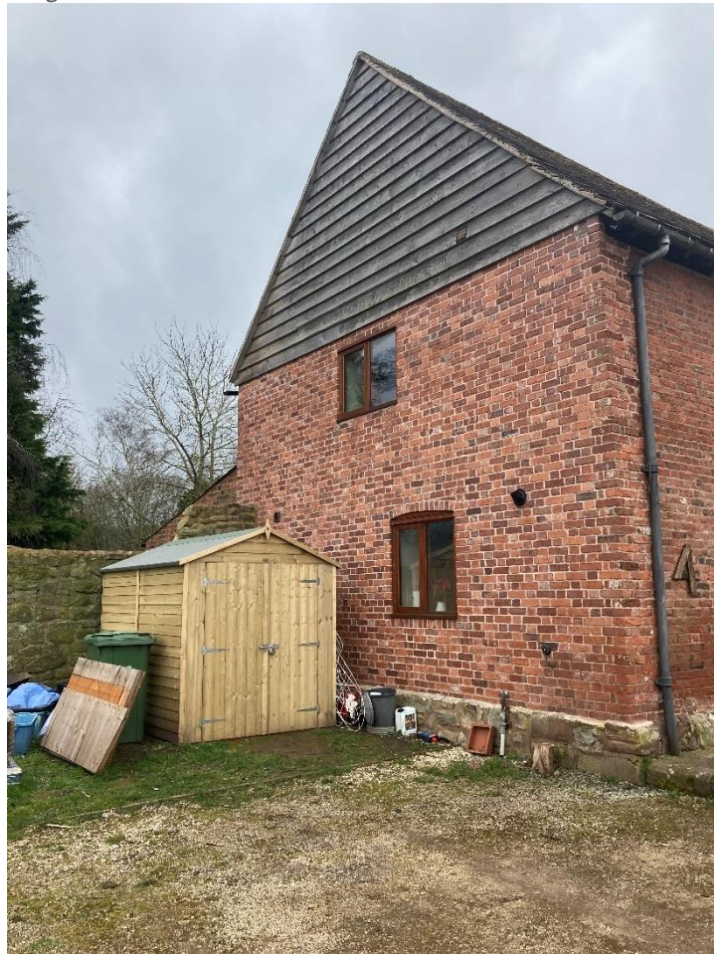
Figure 9: Rebuilt Gable End
