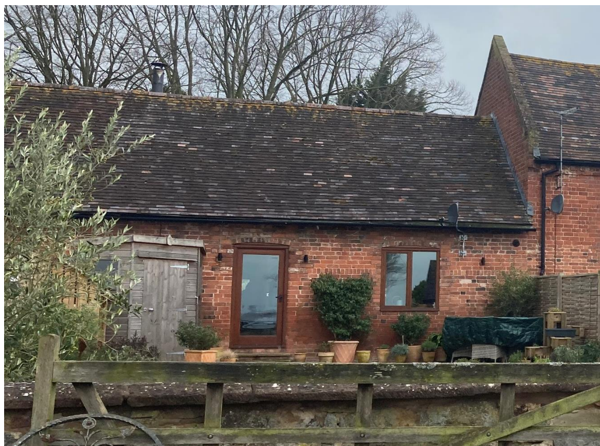
Figure 10: Timber Frame Fully Glazed Door in Arch Header of Adjoining Barn Conversion
