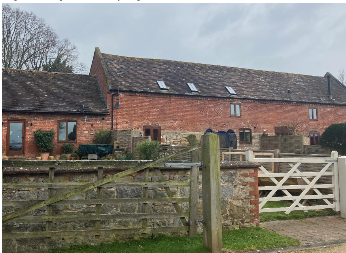
Figure 8: Rooflights visible on adjoining converted barns
