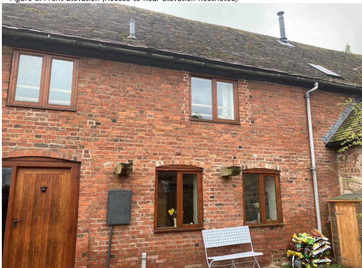
Figure 6: Front Elevation (Access to Rear Elevation Restricted)
