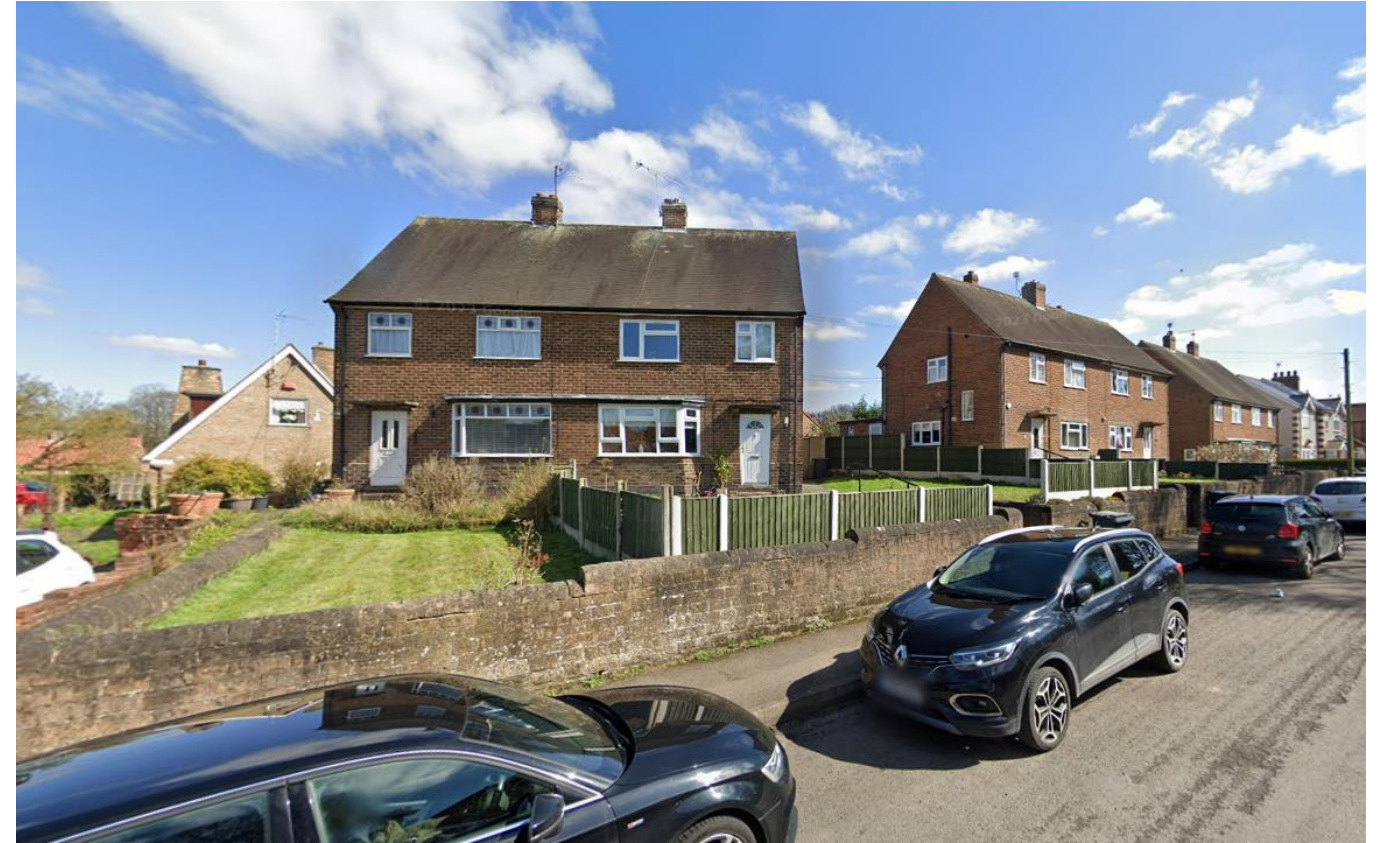
Figure 18 – Existing Houses – 1-11 Church Lane
