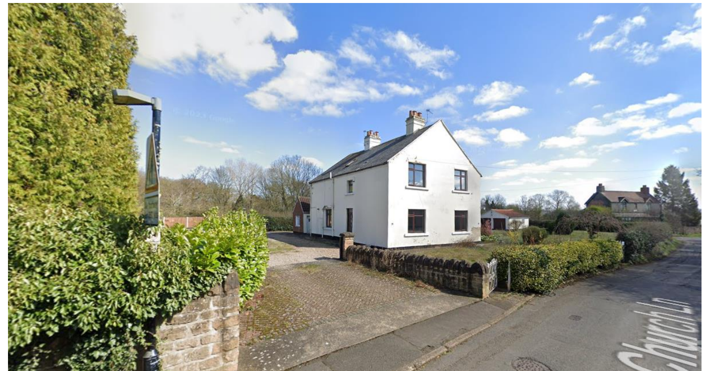
Figure 04– Surrounding Site Photo – Church Lane (South East camera View).
