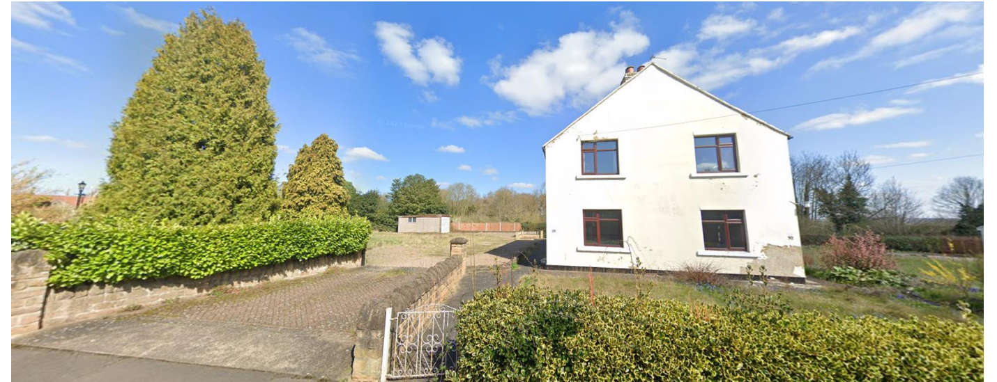
Figure 03– Site Photo – Existing Site entrance to be demolished.
