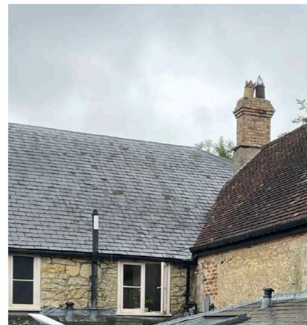
E - Existing slate and hung clay tile
