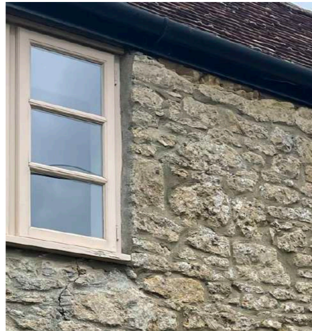
A - Existing rubble stone from original farm house
