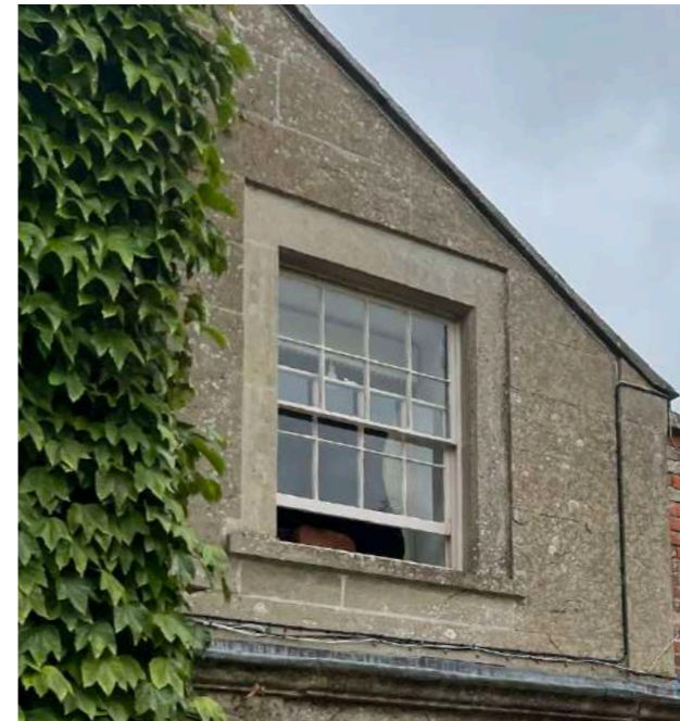
B - Stone blockwork from Georgian extension
