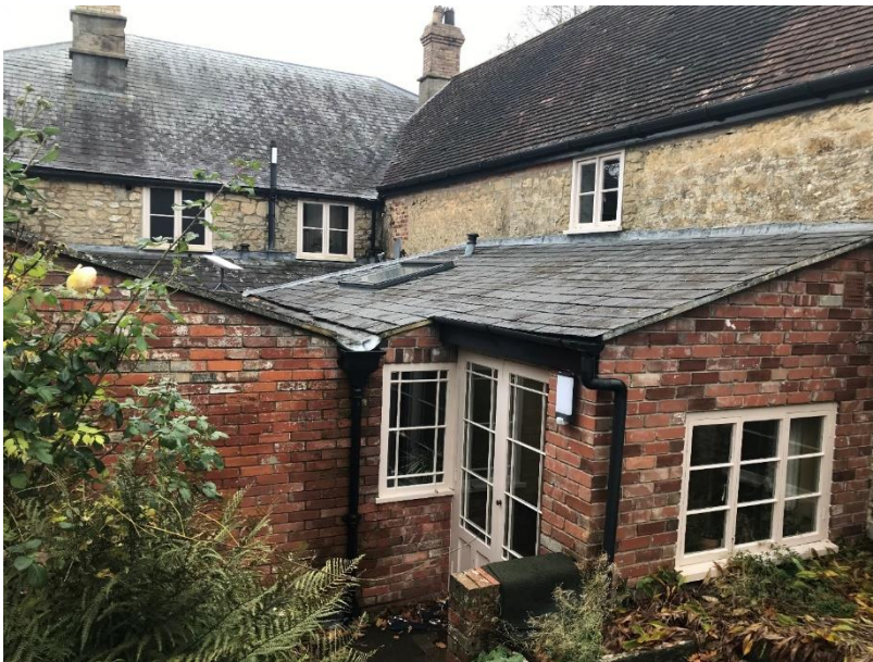
Figure 22 – Within the walled courtyard modern infill structures have been added.
