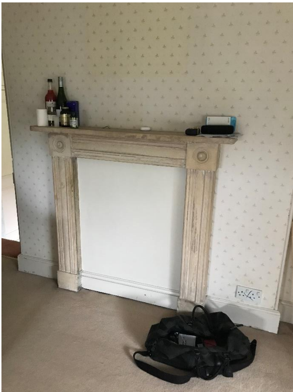
Figure 30 – Some historic features survive at first floor level including fire surrounds in the front rooms.
