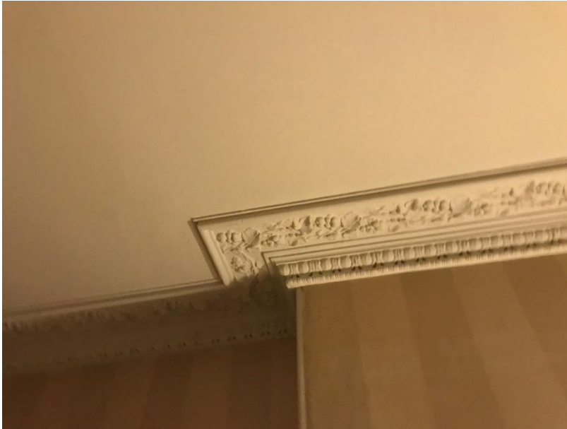
Figure 25 – Some historic cornicing also survives in the 19 th century range; this example survives in the front eastern ground floor room.
