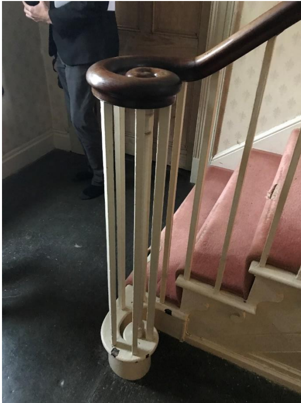
Figure 24 – The historic staircase remains in the 19 th century range.
