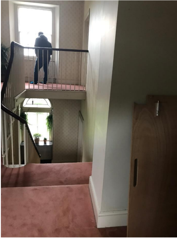
Figure 29 – View from the original range looking toward the front of the Georgian range.
