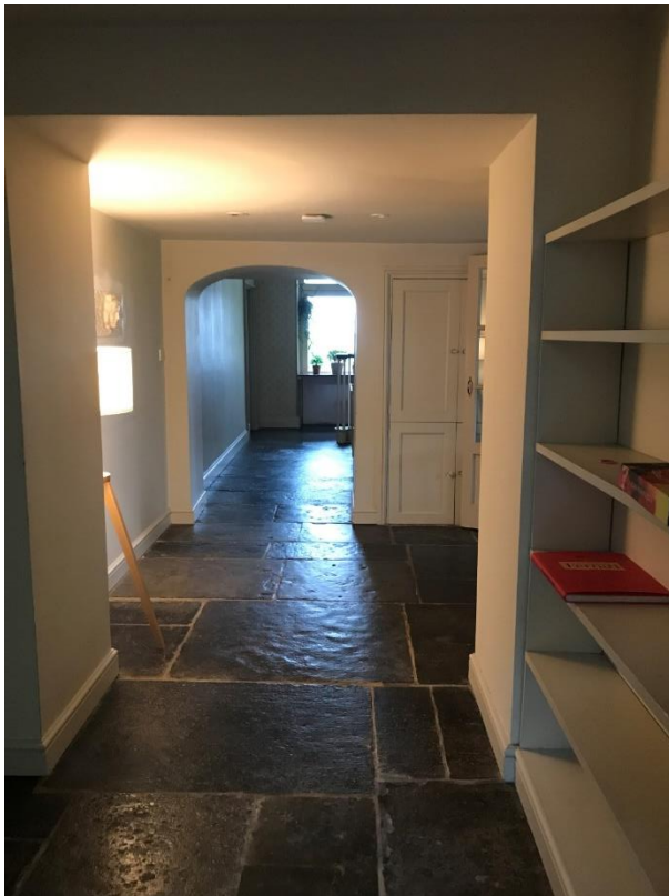
Figure 26 – In the earlier range the floors are a mix of historic and false flagstones.
