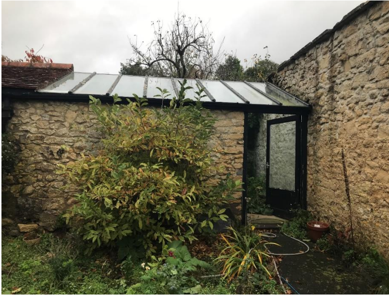
Figure 23 – The historic courtyard wall can still be seen, and a greenhouse has been added into the north of the space.
