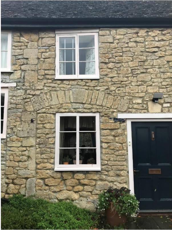
Figure 19 – View of the original range. The access door is traditionally designed, but the stonework suggests that alterations have been made to the access into the property.
