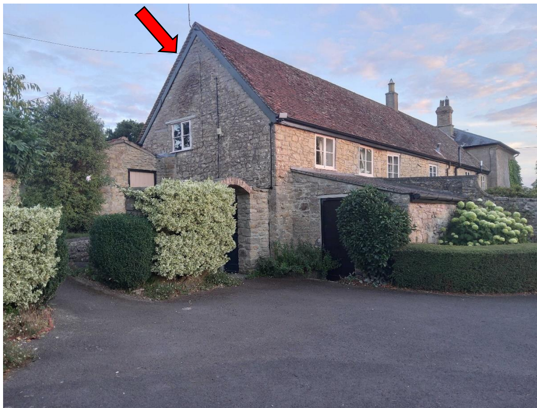
Figure 1: The northwest aspect of B1. The red arrow denotes the emergence location of two common pipistrelles from underneath a tile.
