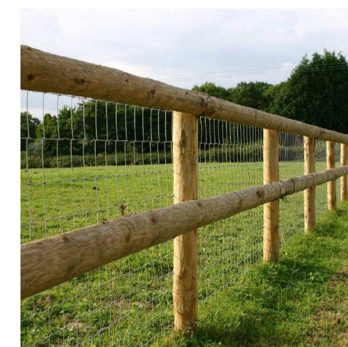
Timber post & rail fence
