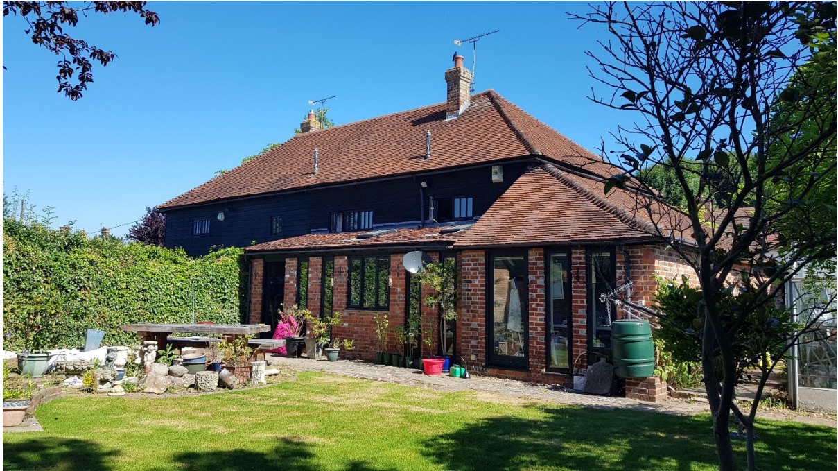
Exterior photograph showing existing rear of property
