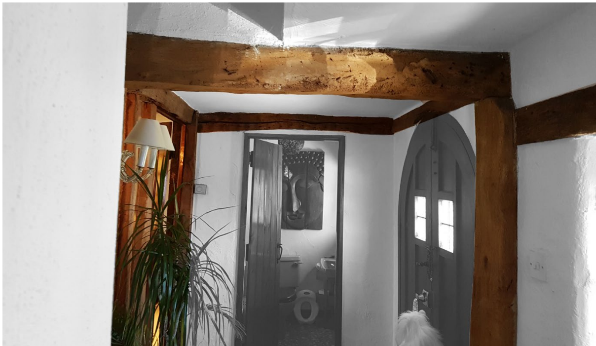
Original Timber Frame Visible Internally
