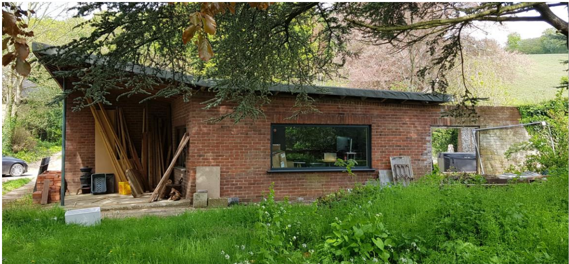
Existing Side Elevation – showing east facing veranda
