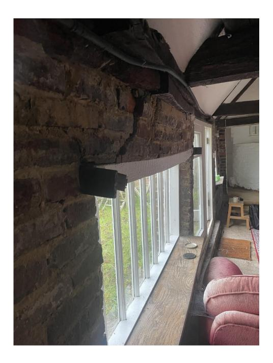
As a separate issue, the timber lintel above the window is undersized causing deflection. There is also evidence of wood boring insect infestation which has weakened the timber.
