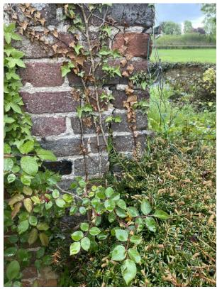
Over the years several areas of lime mortar have been replaced with sand and cement. This should be carefully removed and replaced with lime mortar.
