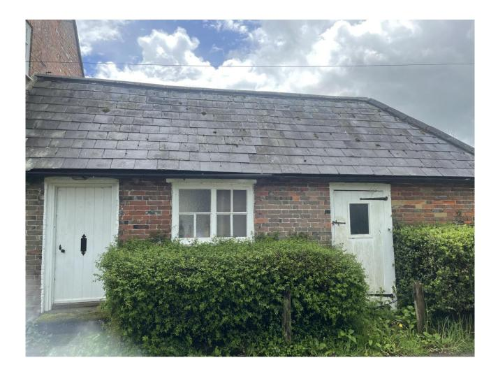
The roof over this area was re-roofed during the 1990/2000 with bitumen BS747 Type 1F roofing felt. The roof to The Forge was re-roofed circa 1970/1980 with a bitumen membrane without hessian strips.
