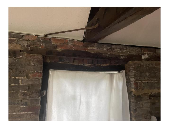
To the rear of the property is a crack in the corner which is evident within the living room which is caused by movement due to the water overflowing from the valley to the main roof.
