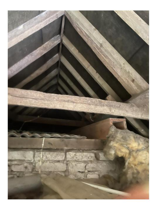
The lathes are machine cut. The lathes are  $\frac{1}{2}$ " x  $\frac{3}{4}$ " untreated which indicates they are from the late 1970's / early 1980's.
