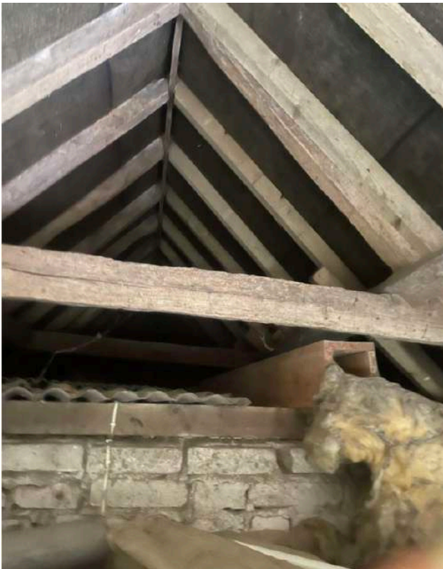
Interior Roof in the barn
