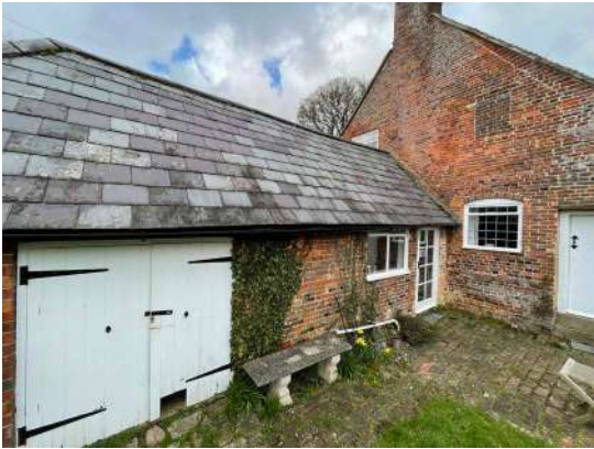
South elevation - The barn joining the main house
