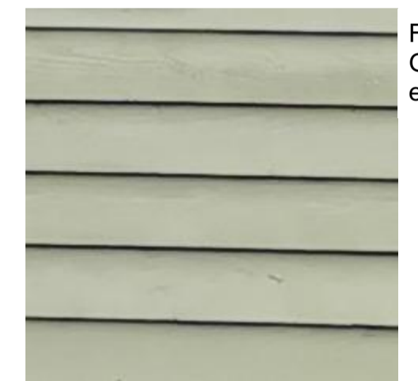
Front Wall and Gable- Timber effect cladding
