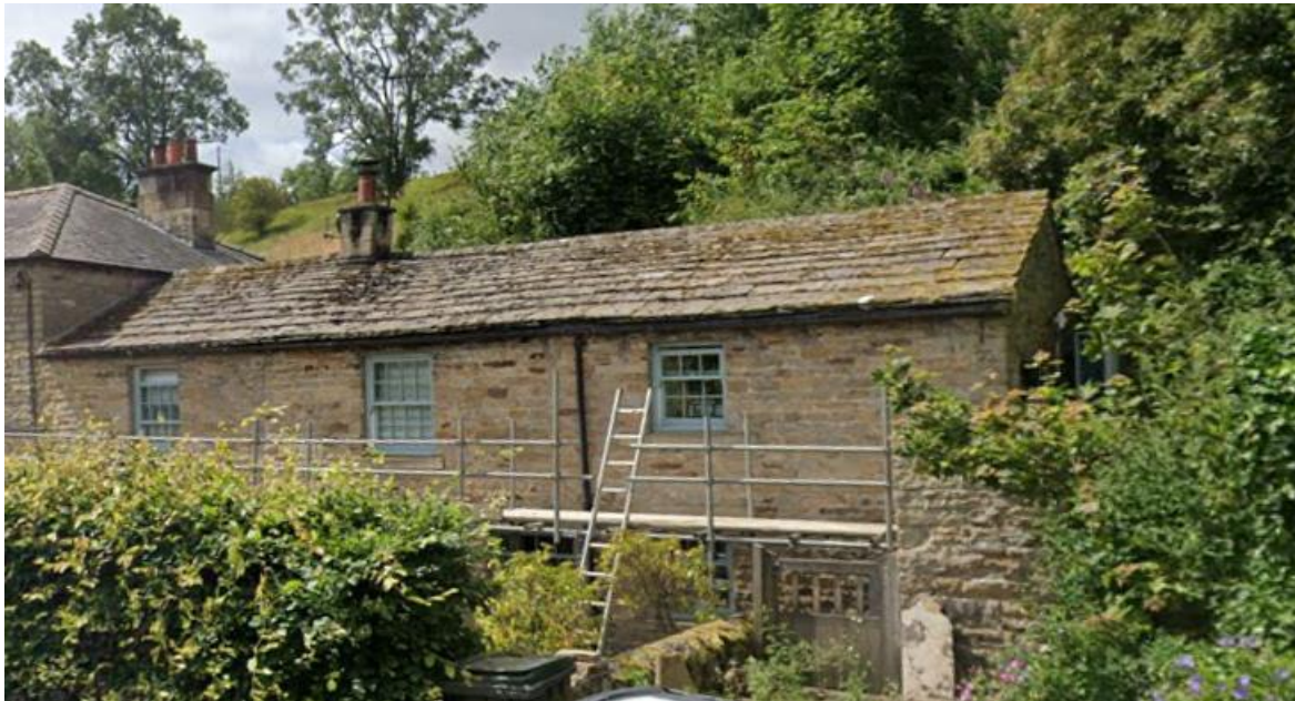
Bridge End Cottage see from the B6297 Road
