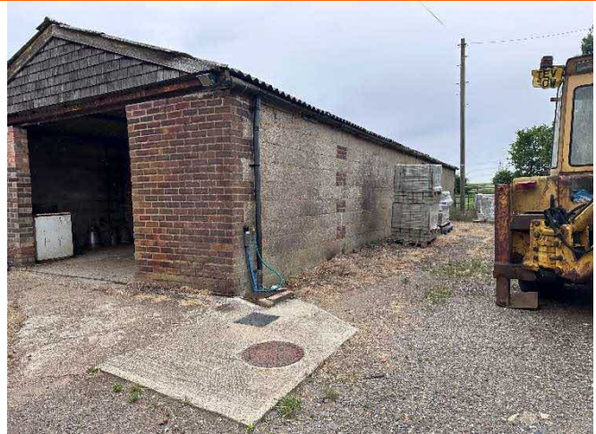
Print 2 View of the barn forming the western section of the site - to be converted
