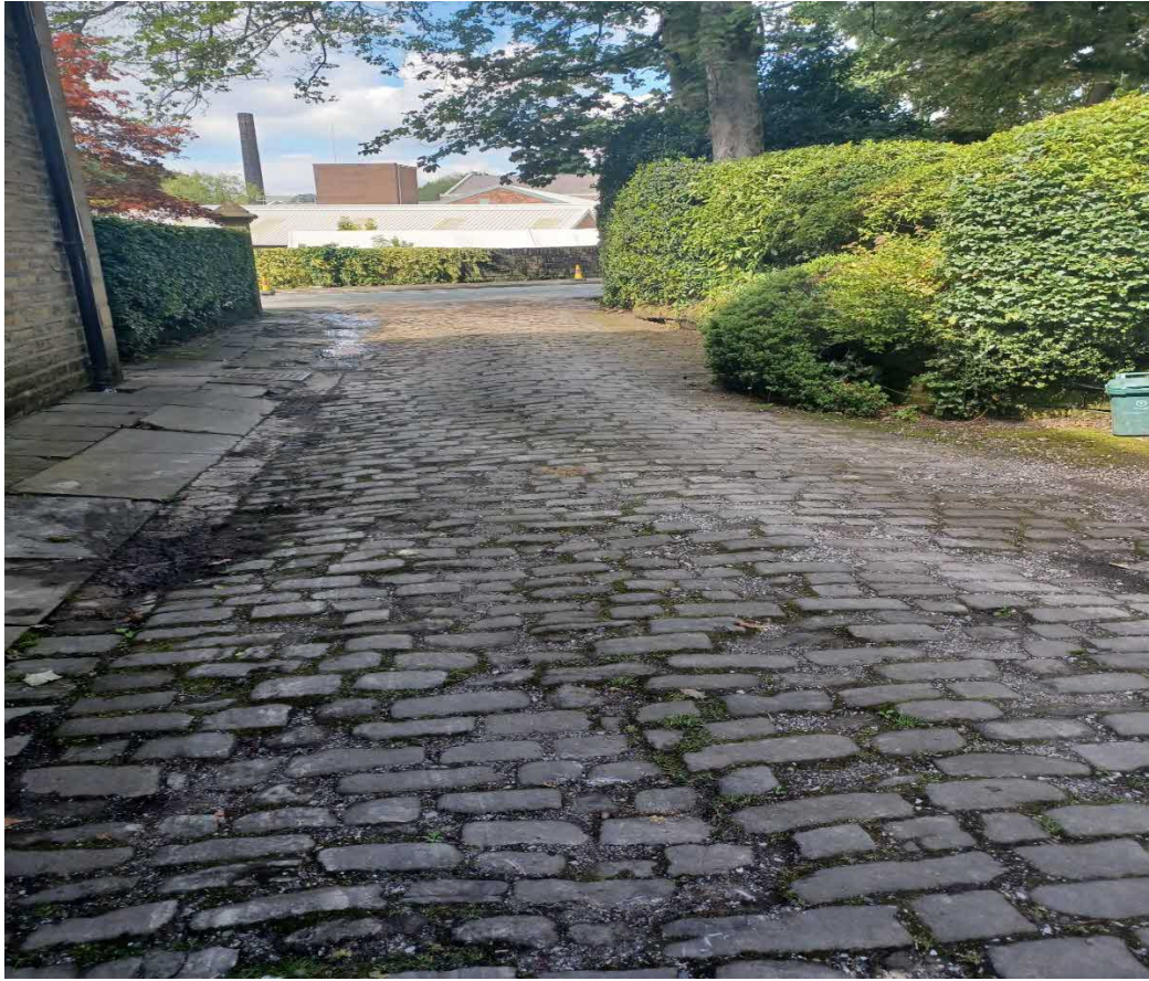
Figure 1 Cobbles to be excavated fronting 1 Delph Lodge (Authors Own, 2023)
