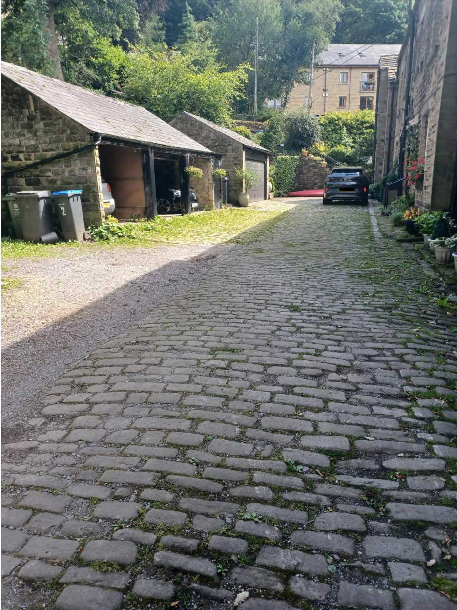
Figure 2 Cobbles to be excavated fronting 2 Delph Lodge (Authors Own, 2023)
