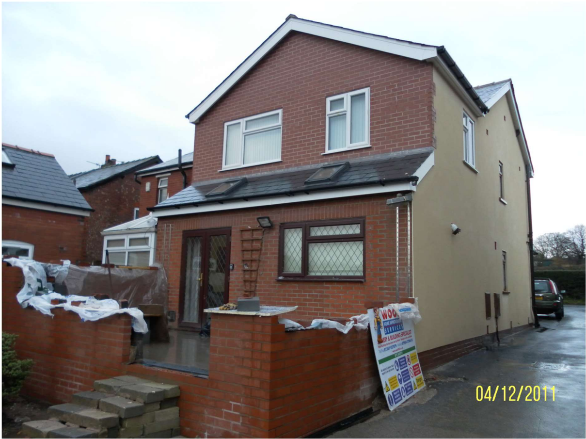
Works commenced on the Conservatory – December 2011
